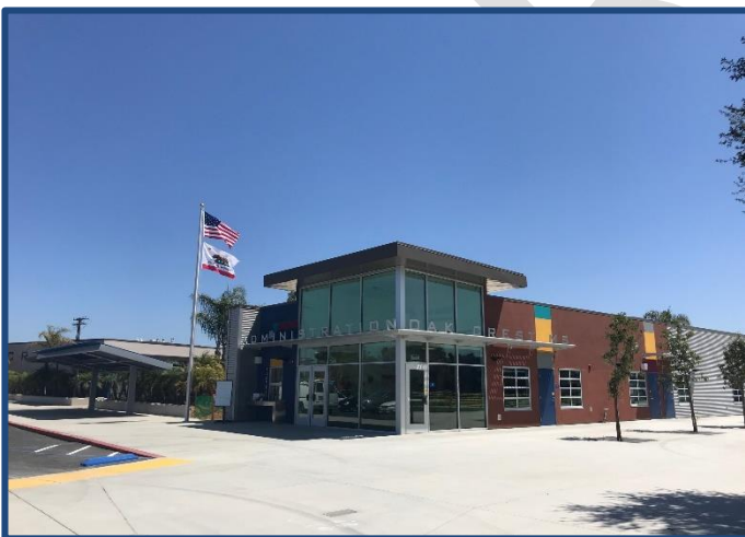
Oak Crest Middle School / Administration Building
