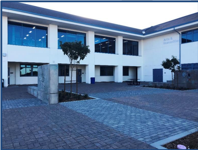
San Dieguito High School Academy Arts & Humanities Building
